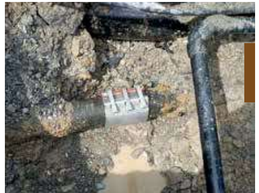
Damaged area on a pipe; quickly and reliably sealed with a STRAUB-REP-FLEX coupling.
