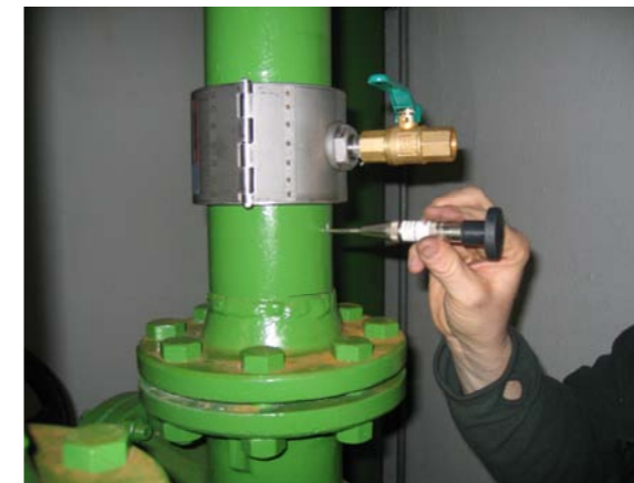
Installation STRAUB-OPEN-FLEX 1L GT
